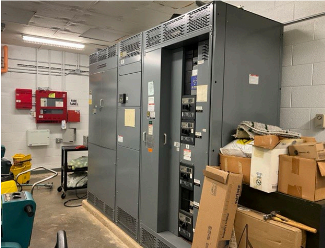
25 - MAIN SWITCHGEAR
