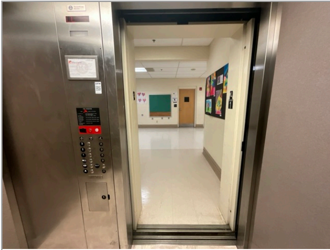
LOBBY LOOKING AT CABS
