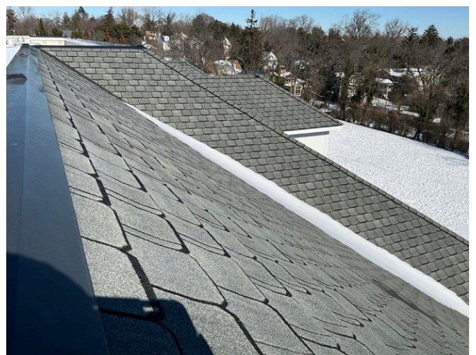
6 - PRIMARY ROOF OVERVIEW
