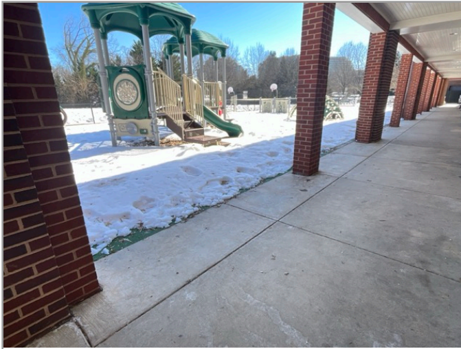
ACCESSIBLE ROUTE TO PLAYGROUND
